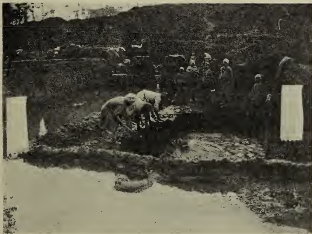
BAILING THE WATER FROM THE PITS INTO THE CANAL
